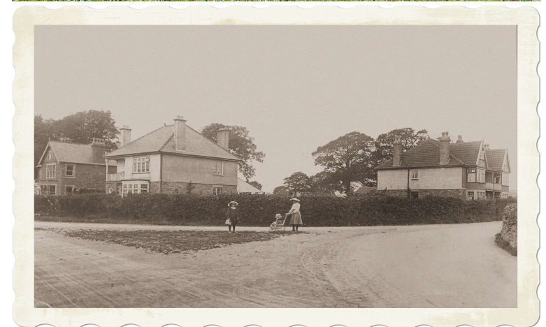
The nearly new Stowell House at about the time of the First World War
