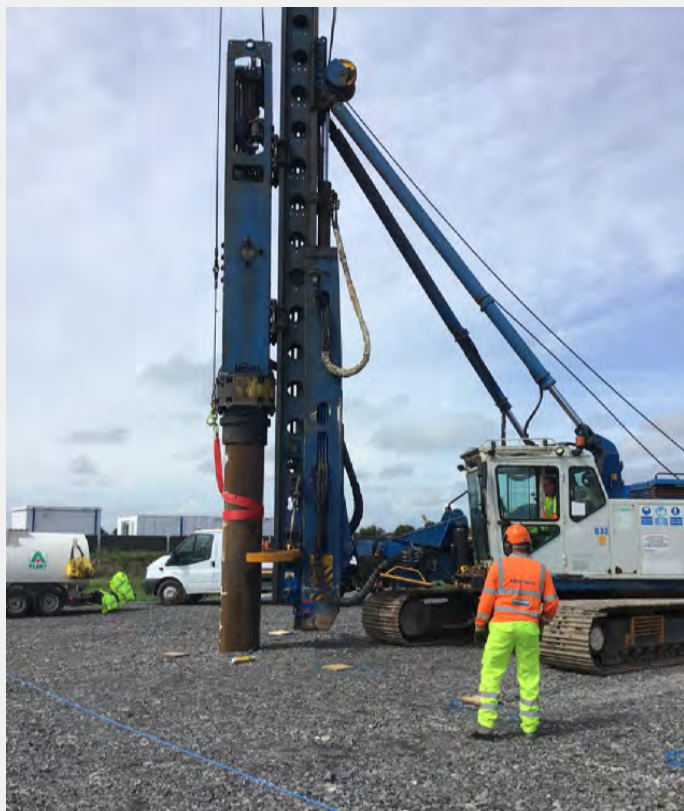
Balfour Beatty's piling rig
