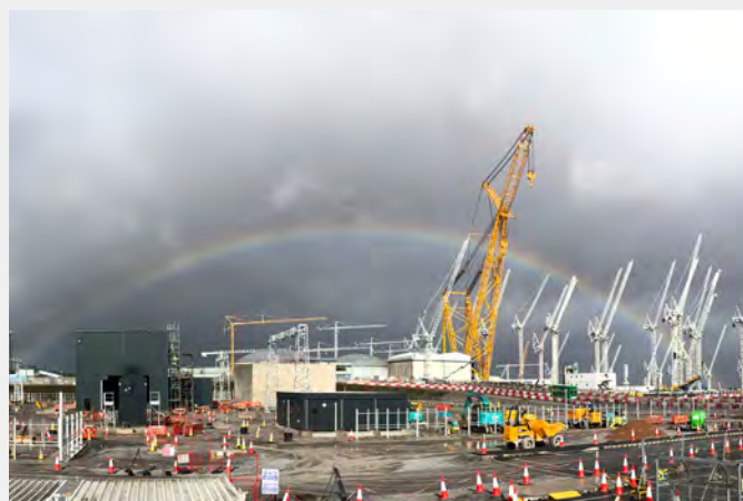
Work is progressing well at Shurton substation
