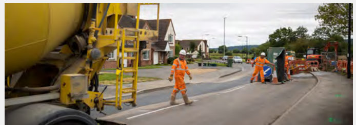
In Nailsea, we're working very close to peoples' homes
