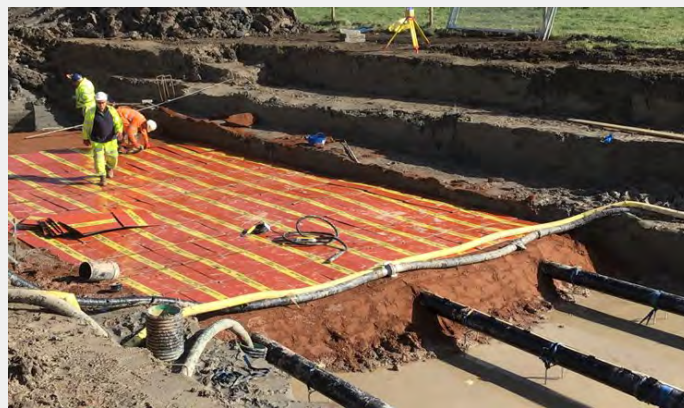
Three cable ducts are laid in each trench
