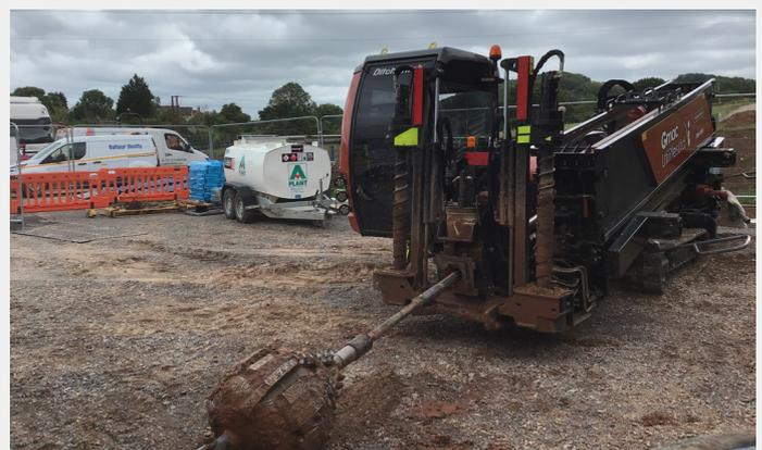
HDD machine for drilling under roads and rivers
