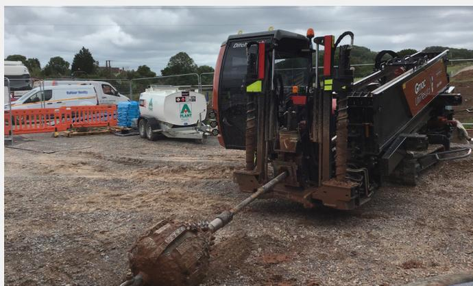
HDD machine for drilling under roads and rivers
